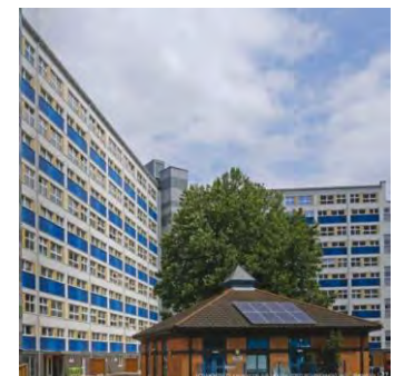
Wilmcote House, Plymouth (Source: ECD Architects)
