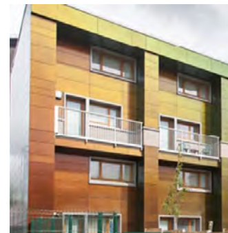
Ernley Close, Manchester (Source: 2e Architects)
