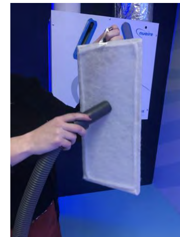
MVHR filters are easy to remove and clean, clean filters improve energy efficiency. (Sources: Vent Axia, Nuaire,)
